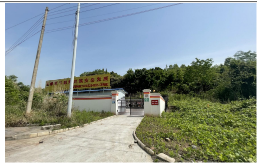
厂区南侧配气站现状
